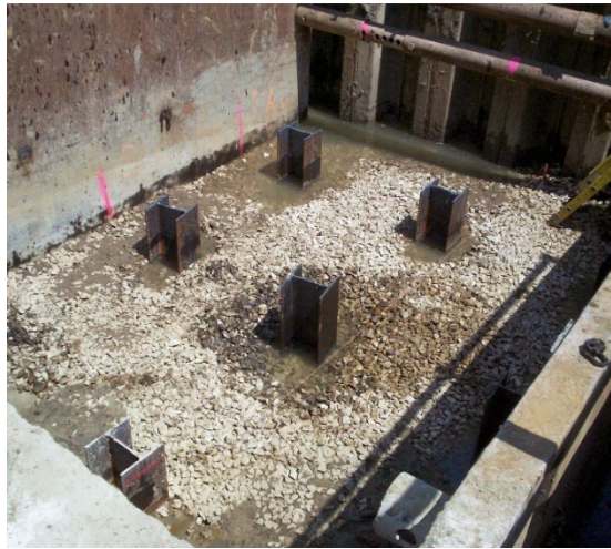
Figure 14. Piles cut-off at plan elevation
